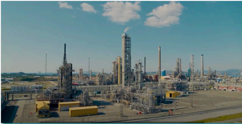
Figure 4.4: CO 2 Technology Center Mongstad, Norway. (Courtesy of Technology Center Mongstad, tcmda.com)
